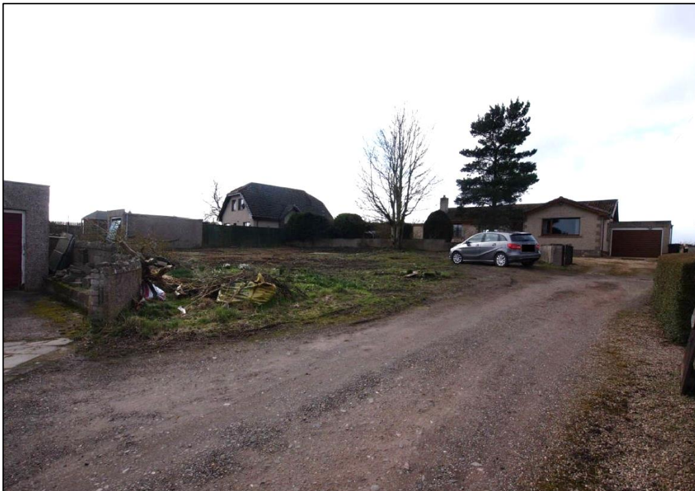
Figure 3: Photograph of site looking east towards Hillcrest. Existing garage is visible to the rear of the site.
